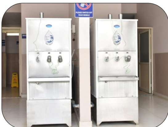
Water Cooler with RO System
